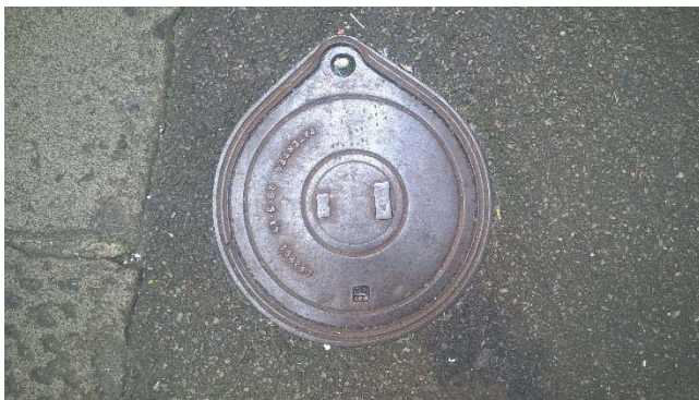
Photograph 9: Potential underground storage tank cap observed on the footpath of Bligh Street within the north west corner of the site.
