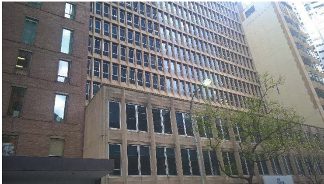
Photograph 1: Current site conditions at 4-6 Bligh Street, Sydney NSW.
