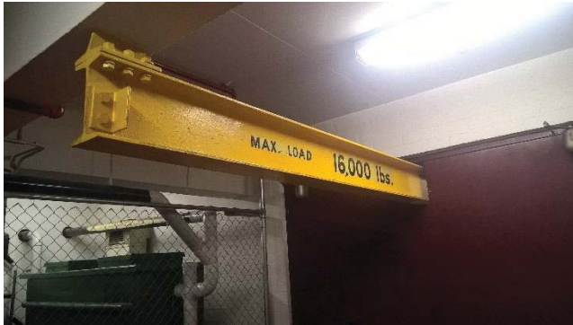
Photograph 3: Possible hoist system observed within the basement car park
